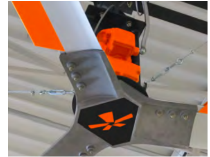
Stepped leading edge creates venting which increases performance.
