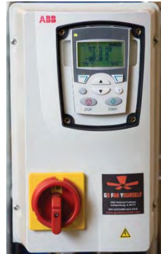
Keypad relocated to 4x4 electrical box
