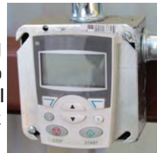
Keypad relocated to 4x4 electrical box
