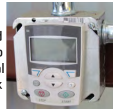
Keypad relocated to 4x4 electrical box
