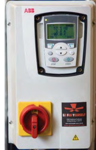
Keypad relocated to 4x4 electrical box
