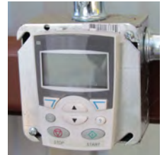
Keypad relocated to 4x4 electrical box
