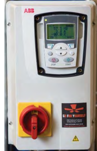
Keypad relocated to 4x4 electrical box
